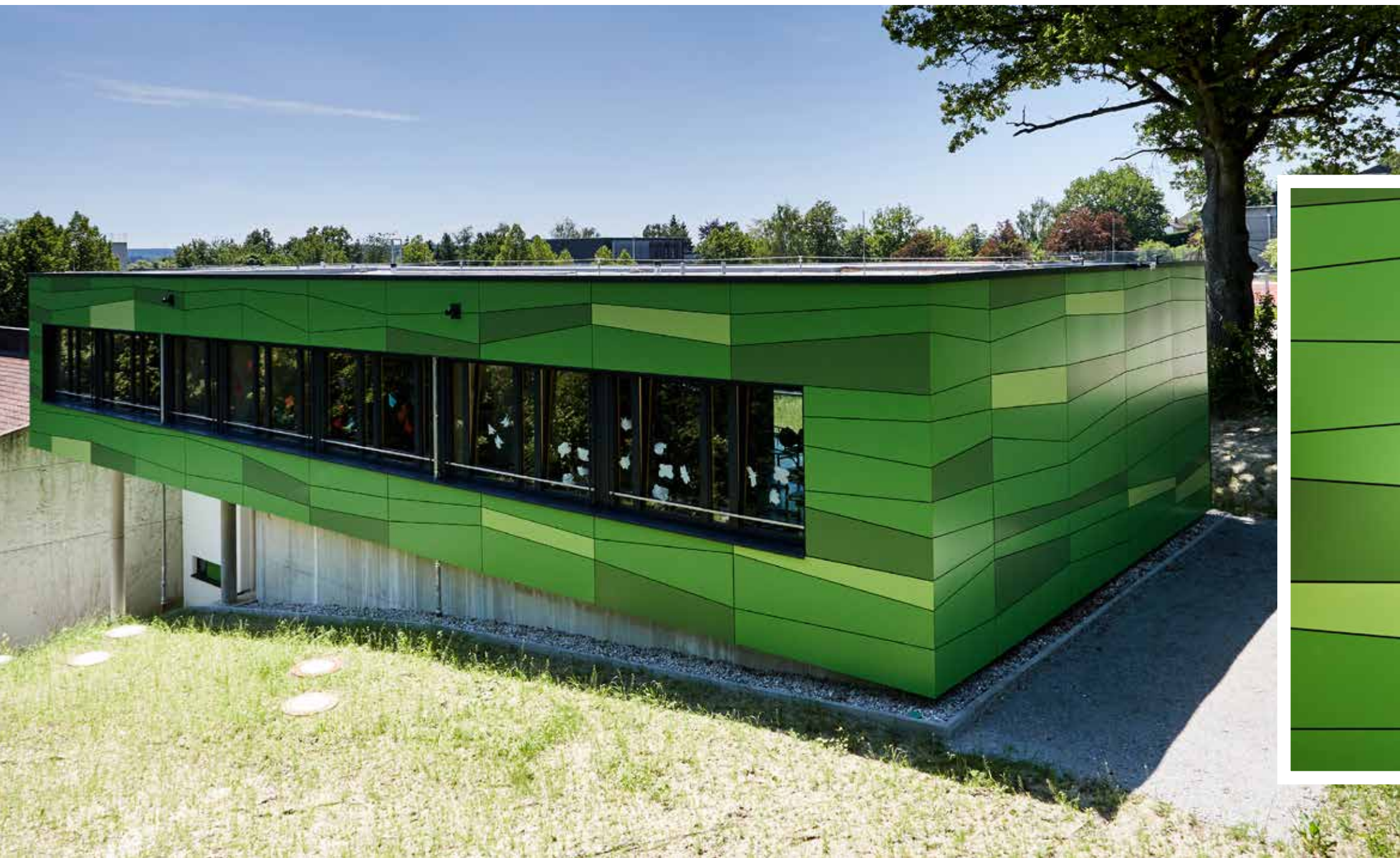
Project: Betty-Greif-School, Pfarrkirchen, Germany
