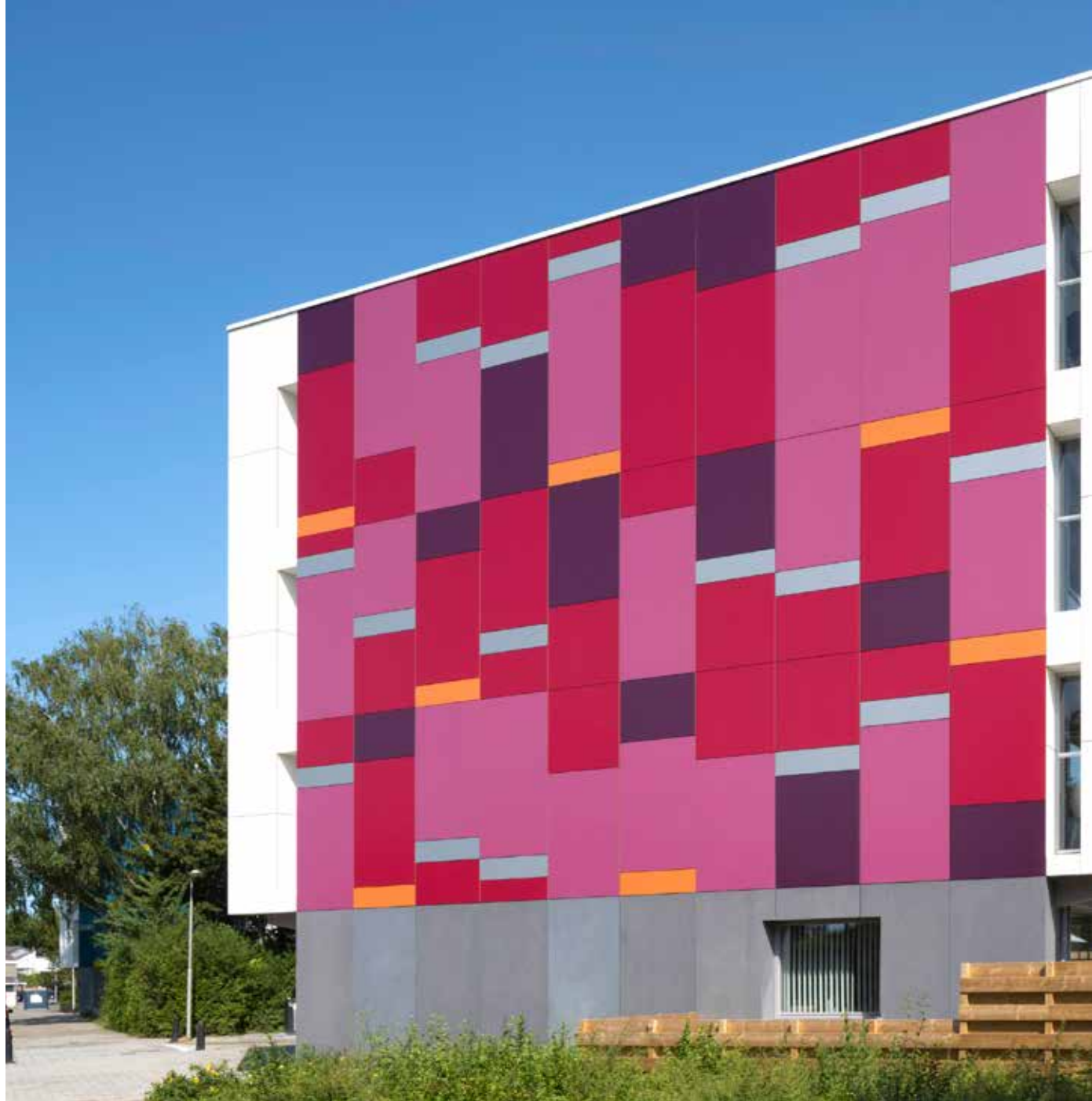
Project: Renovated flats, Emmeloord, The Netherlands
